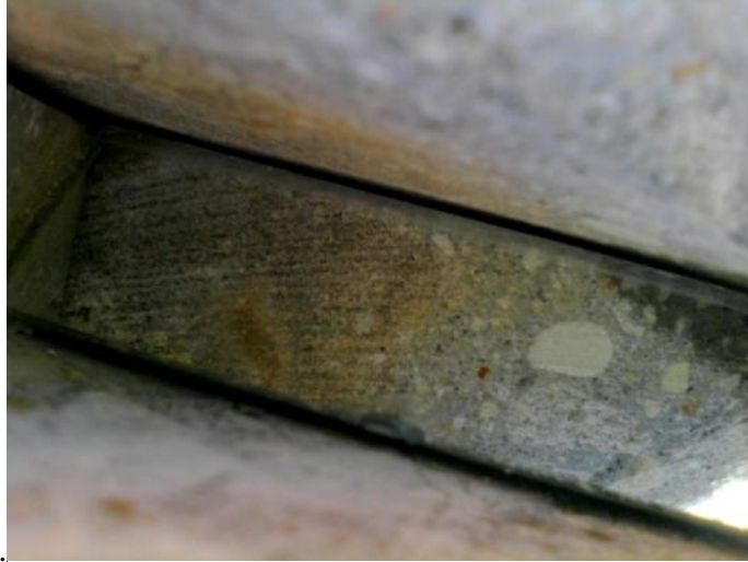
Figure 24 - Field Image from Joint Inspection Device
