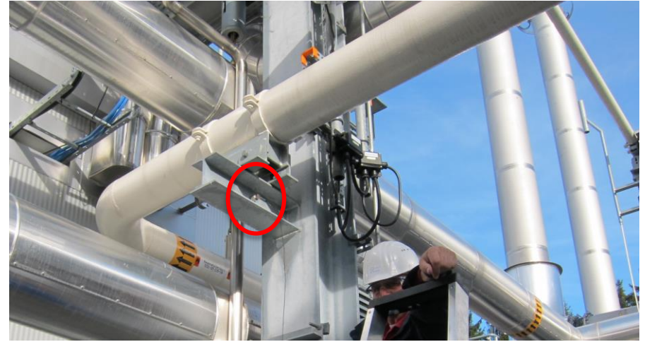
measurement on support beam
