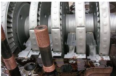
Figure 6 - New Current Diaphragms in the Turbine Case
