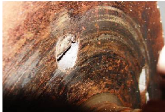
Figure 3- Severe Disc #4 Damage: Rubbed Metal Filled Equalizing Holes
