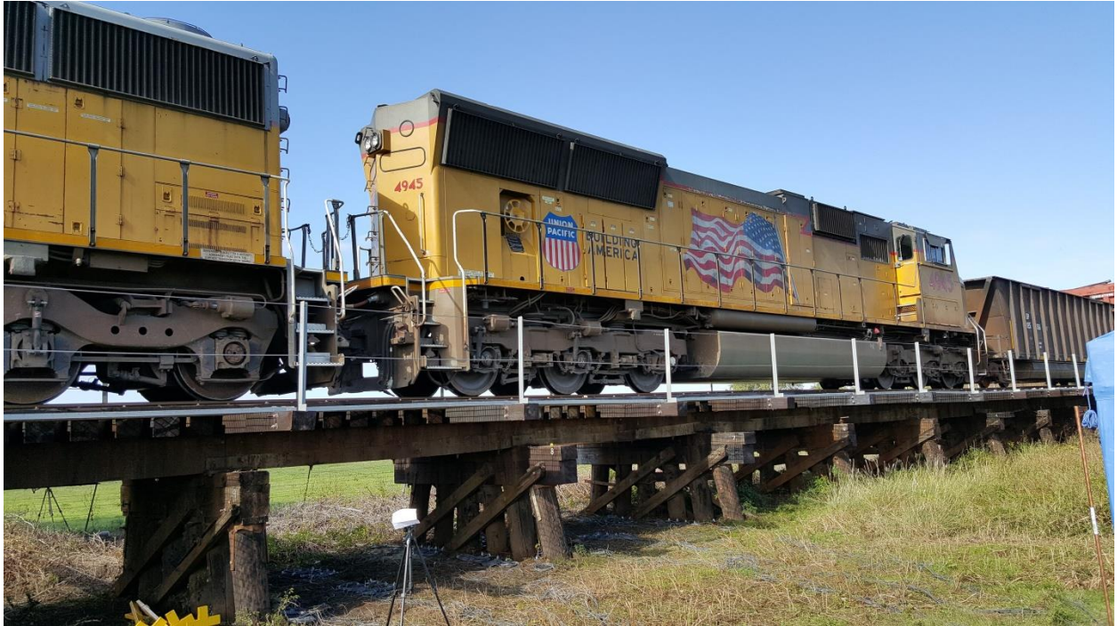
Figure 14. Train over Bridge 17.14 during test
