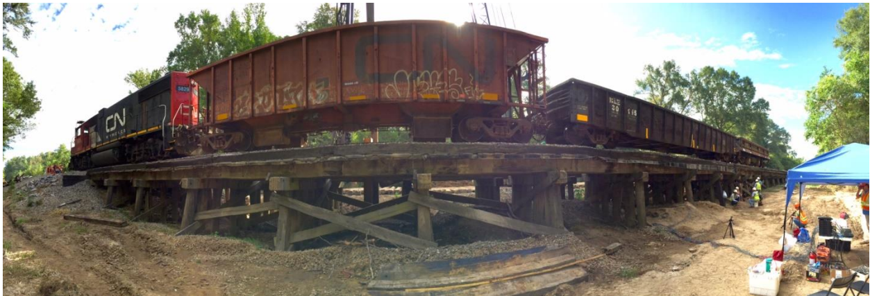
Figure 10 - Train over Bridge 816.9 during test
