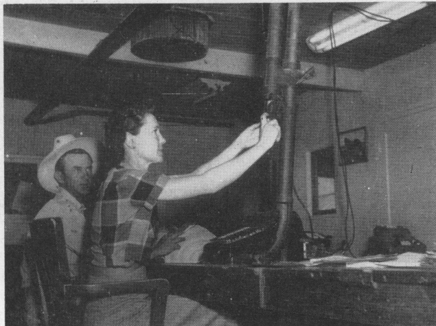
Figure 23. Office on a Texas livestock auction market. A pneumatic tube is used to bring sales tickets into the office from auctioneer's box.
