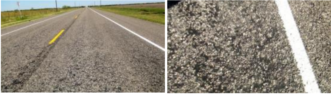
Figure 29. Example of Inadequate Performance— 16-CRP-2, Post First Winter.
