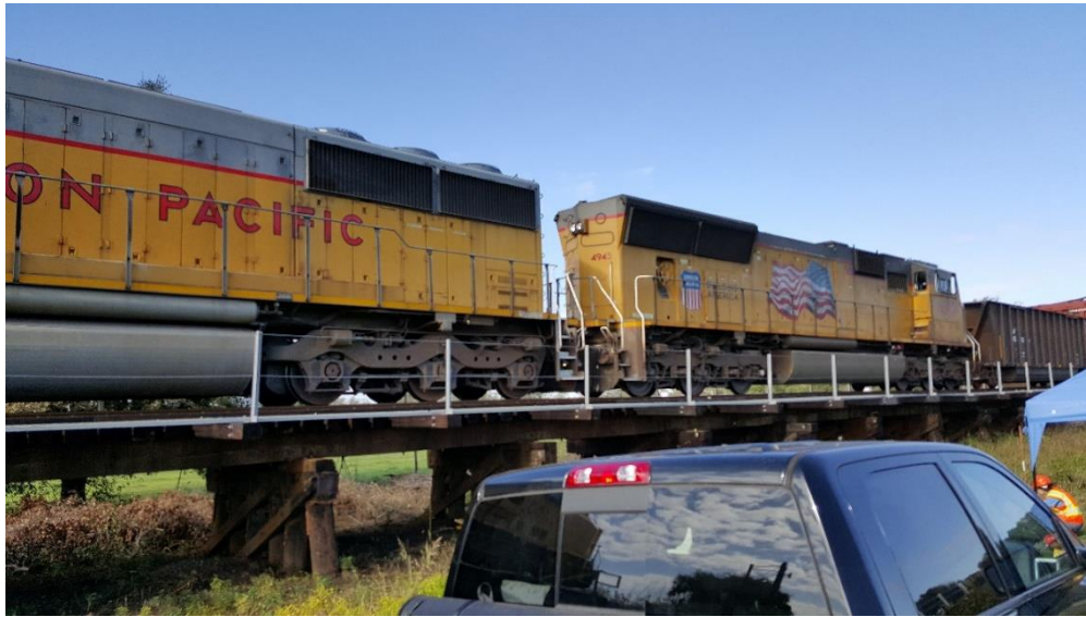
Figure III-2: Work Train Crossing Bridge 17-14
