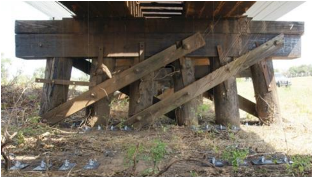
Figure III-7: String Potentiometer Setup Under Span 7
