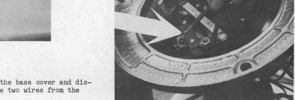
2. Removing the base cover and disconnecting the two wires from the terminals.
