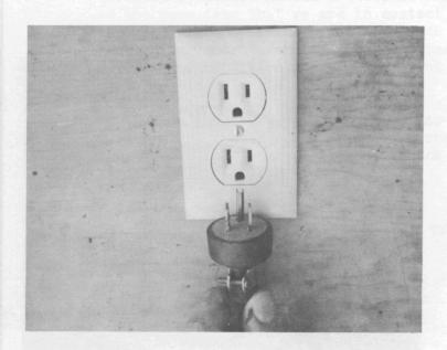
6. A 115-volt grounded duplex outlet with three-prong grounded plug being connected.
