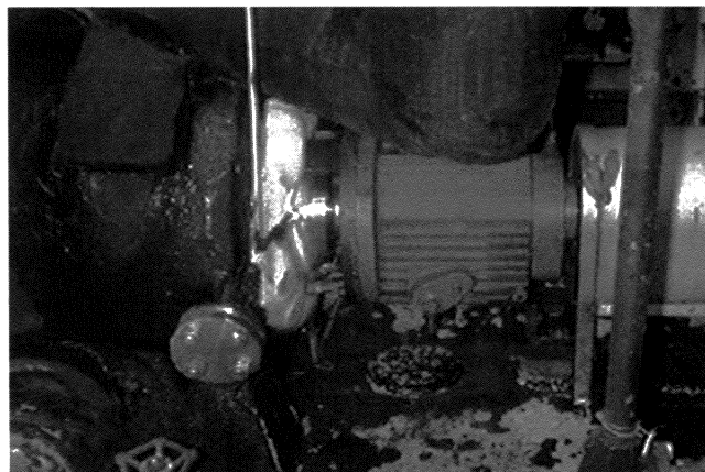
Figure 8. Dual Nonpressurized Seal Installation at the Plant.
