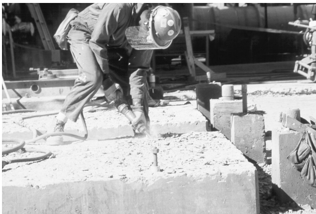
Figure 22. Chipping of Concrete Foundation.
