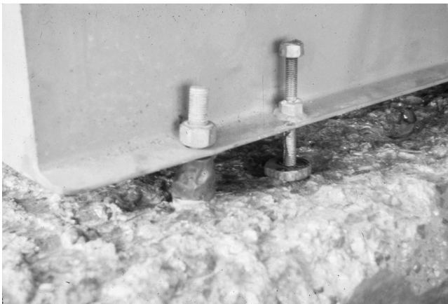
Figure 10. Anchor Bolt and Jack Bolt System.
