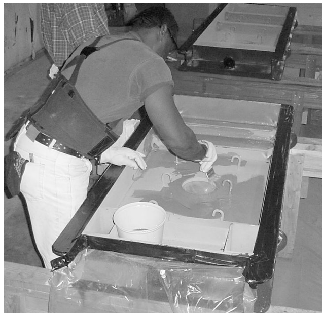
Figure 13. Epoxy Bond Adhesive for Cementitious Grout.
