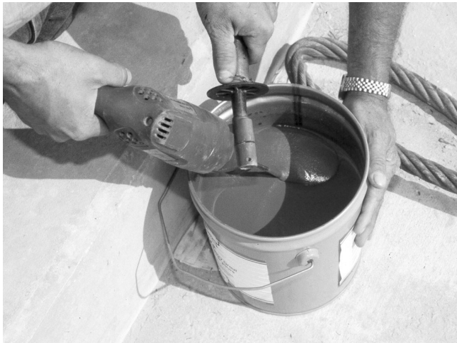
Figure 21. Mixing of Low Viscosity Epoxy Grout.
