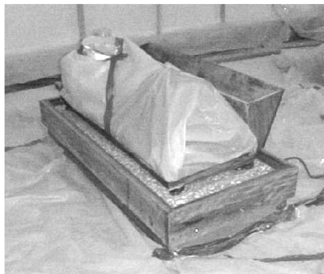
Figure 19. Pregrout Installation Using Conventional Method.
