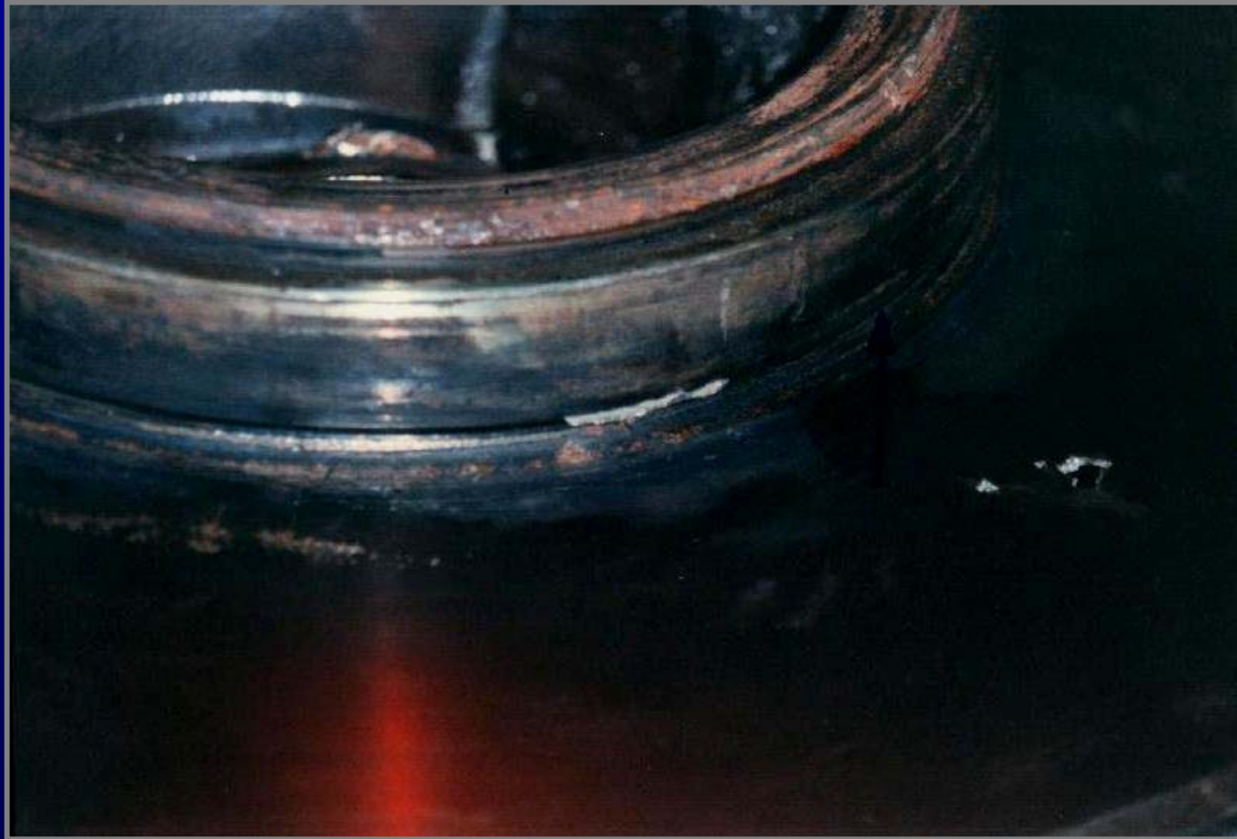
SEVERE RUBBING AT WEAR RINGS - 1996
