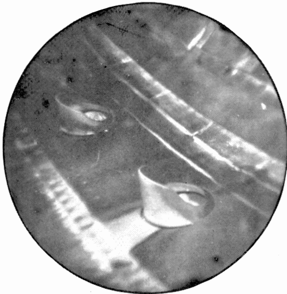
Figure 21. Boroscope view of Combustion Equipment.
