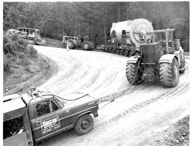
Figure 11. Transporting the 166 Ton Geysers Unit 13 Generator Stator Up Steep Mountain Roads to the Plant Site.
