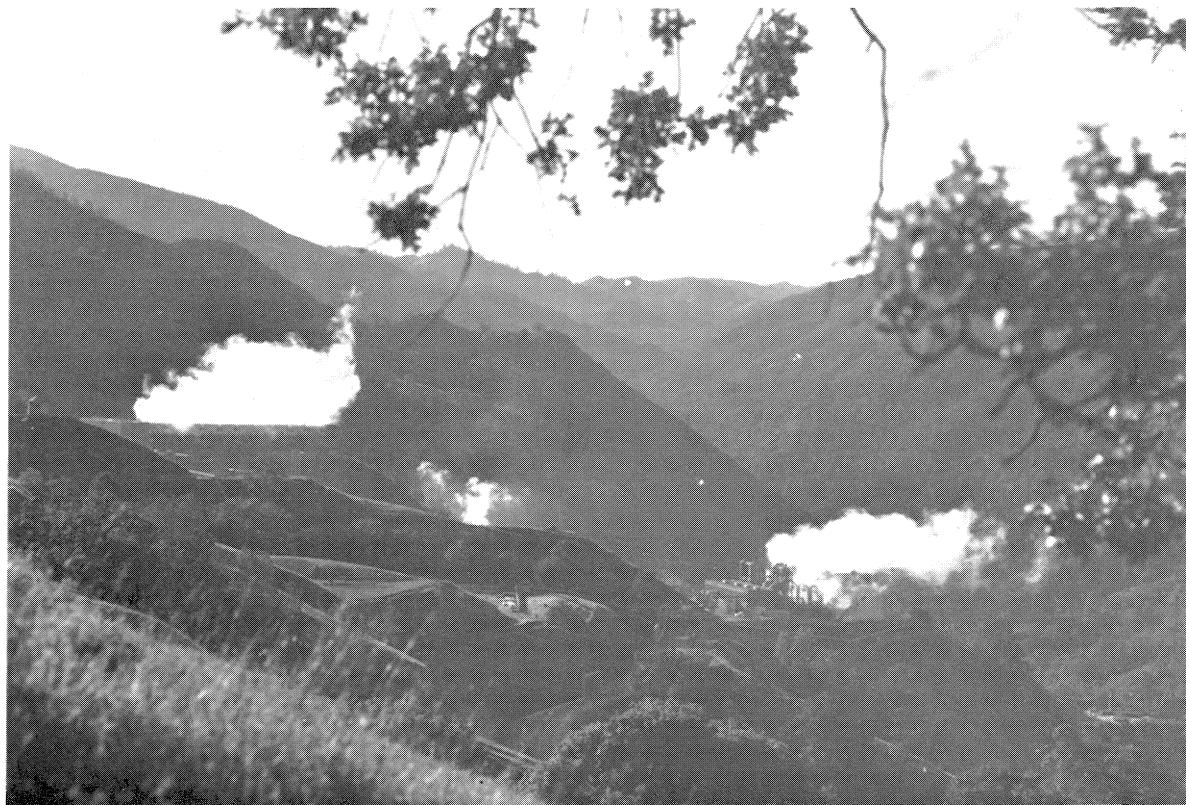
Figure 10. Mountainous Terrain of The Geysers Power Plant with Units 5 and 6 on the Left and Units 3 and 4 on the Right.
