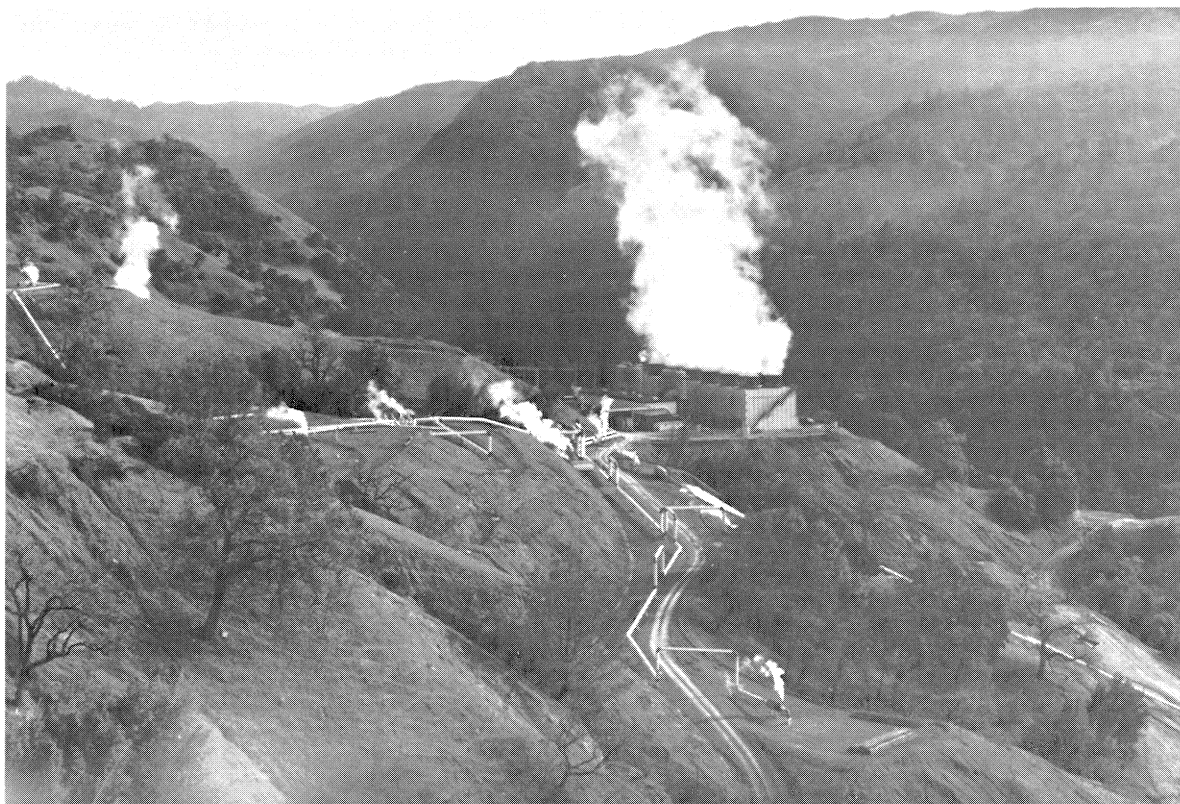
Figure 9. Geysers Units 3 and 4 Showing Steam Gathering System with Expansion Loops.
