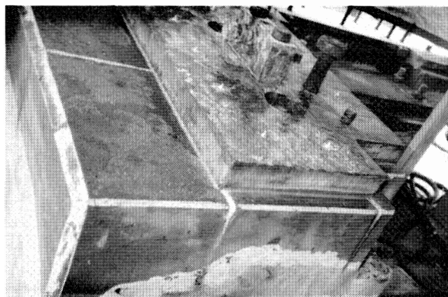
Figure 26. Regrouted Sole Plates in Field-Turbine and Compressor.
