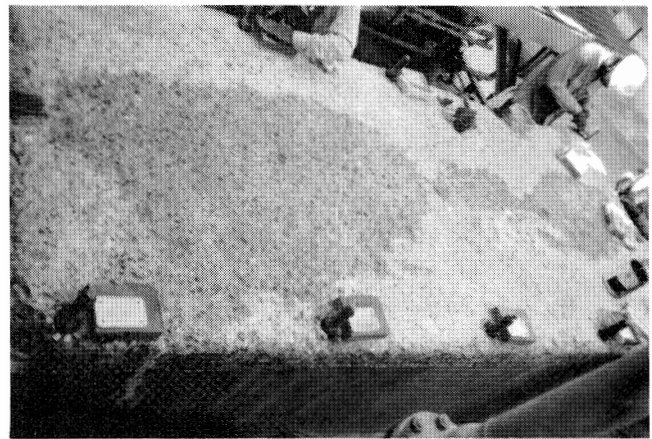
Figure 1. Concrete Mezzanine Base Prepared for Baseplate.
