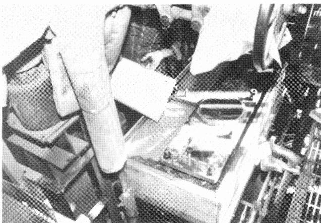
Figure 43. Grout Being Poured from Only One Side of the Forms.
