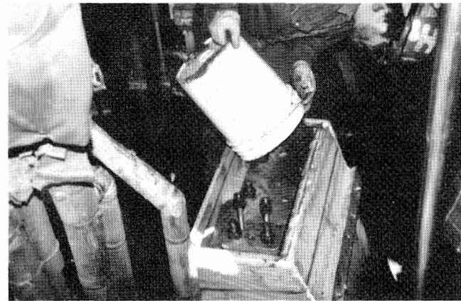
Figure 45. Grout Again Being Poured So It Could Flow under the Rails.
