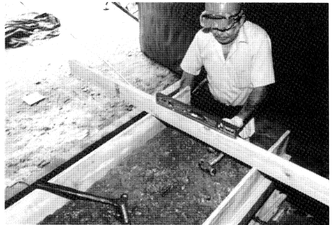
Figure 31. Grout Forms Constructed around the Compressor Outboard Soleplate.
