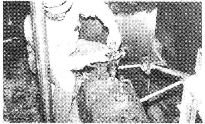
Figure 29. Die-Nut Used to Chase the Anchor Bolt Threads.
