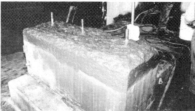
Figure 28. Epoxy Primer Coating Placed on the Clean Concrete.
