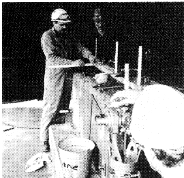
Figure 34. Soleplate Being Positioned in the Horizontal Plane.
