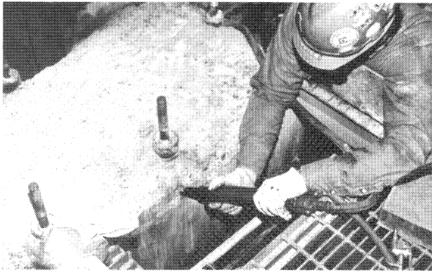
Figure 27. Chipping Away of the Oil Stained Concrete.
