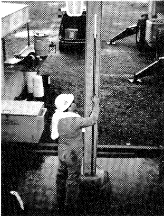
Figure 4. Benchmark Determined for Optical Alignment.
