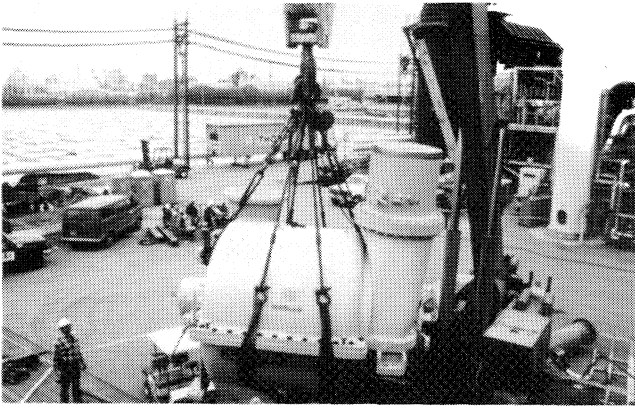
Figure 53. Compressor Being Lifted into Place.
