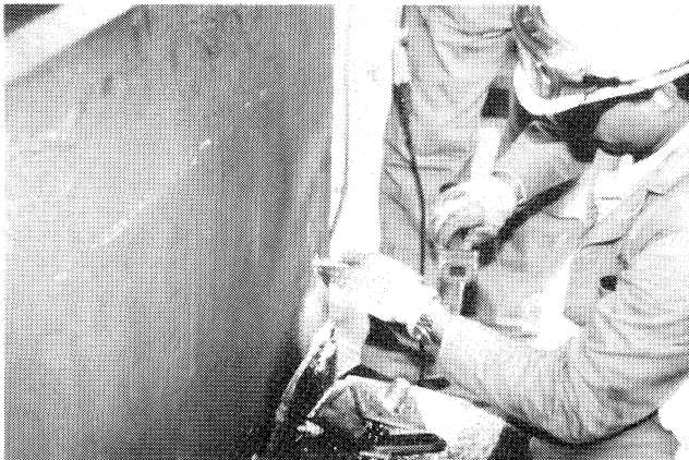
Figure 9. References Established on the Soleplates.
