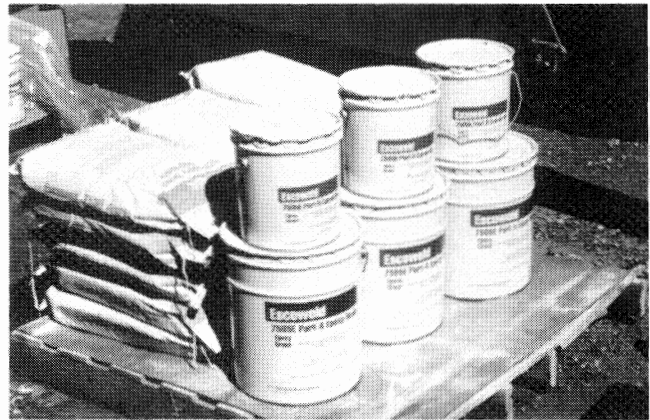
Figure 39. Grout Material Staged by Volumetric Unit.
