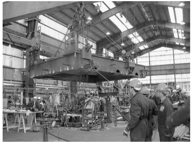
Figure 35. Baseplate Removed from Foundation.
