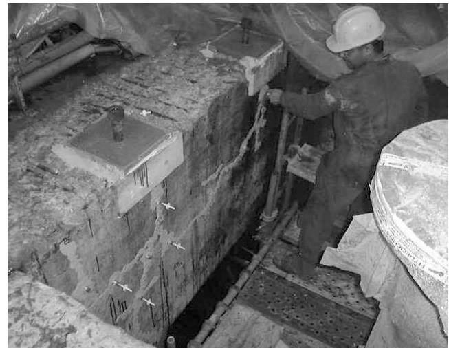
Figure 37. Foundation after Repair.
