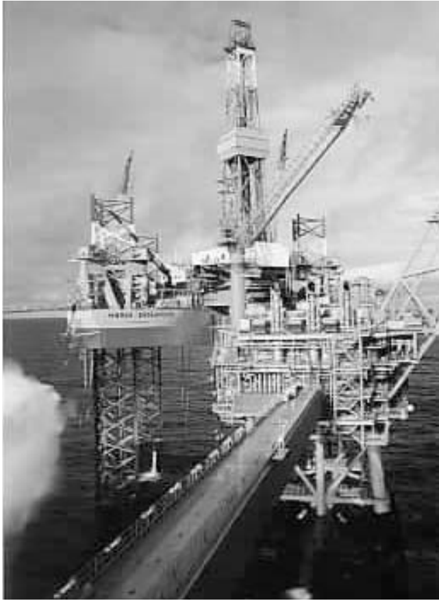
Figure 7. Offshore Platform Where Turboexpander Is Installed.
