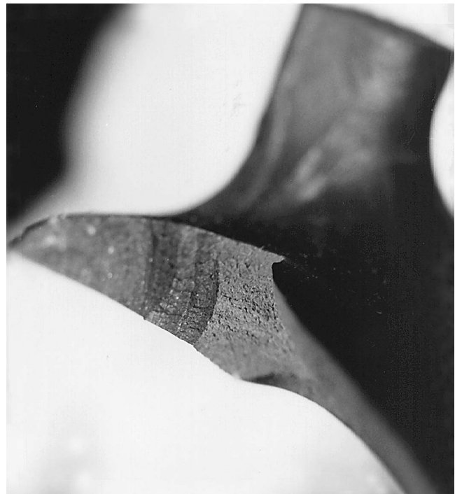
Figure 6. Combination of Pitting, Corrosion Fatigue, High Cycle Fatigue in Low Pressure Blade Airfoil Section.
