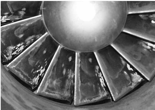
Figure 22. Impeller Inducer Just after Cleaning, but before Heavy Erosion.
