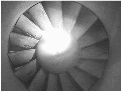
Figure 18. Normal Dirt Buildups on Impeller—Vibration Can Move Up and Down Somewhat Depending on How Dirt Sheds. Impeller Still in Good Shape Here.
