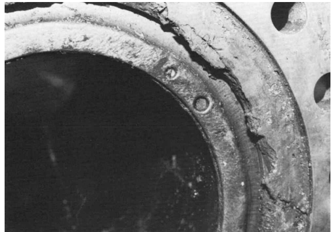
Figure 25. Sludged-Up Continuous Lubed Coupling.
