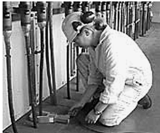
Figure 3. Clip-on CT Around Supply Cable.
