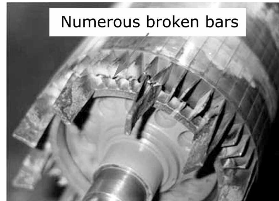
Figure 9. Crane Motor—Broken Rotor Bars.
