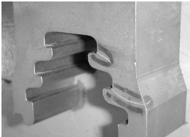
Figure 1. Magnetic Flux Inspection of a Cracked Blade Root.
