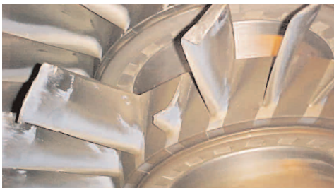
Figure 10. Axial Air Compressor Blade Failure. The Second in the Compressor's 22 Year Operating History.
