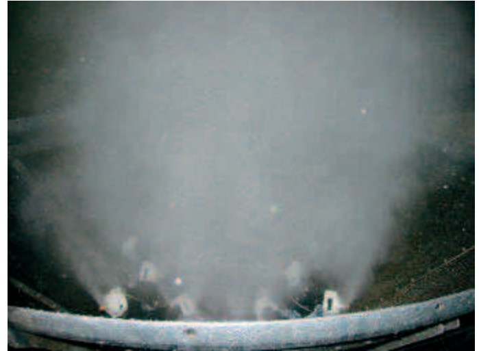
Figure 2 Water wash manifold with 12 nozzles giving 25 \mu\text{m}_{\text{VMD}} droplets at 4.4 l/min
