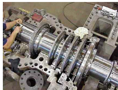
Figure 7. Installation of New Steam Path.
