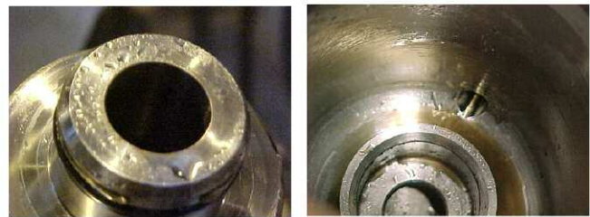
Figure 3. Liquid Accumulation in Particulate Filter Housing.
