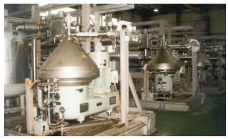
Figure 37. Two-Stage Centrifugal Fuel Treatment Plant for Heavy Fuel Oil. (Courtesy Westfalia Separator)
