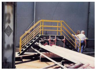
Figure 45. Poor Design of Piping from No. 2 Diesel Fuel Tank.
