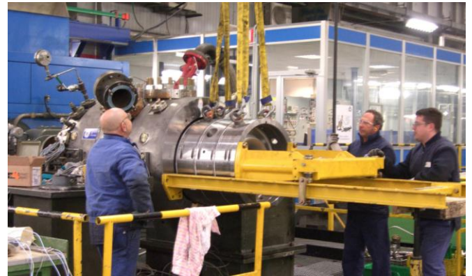
Figure 27. HP bundle removal after MRT
