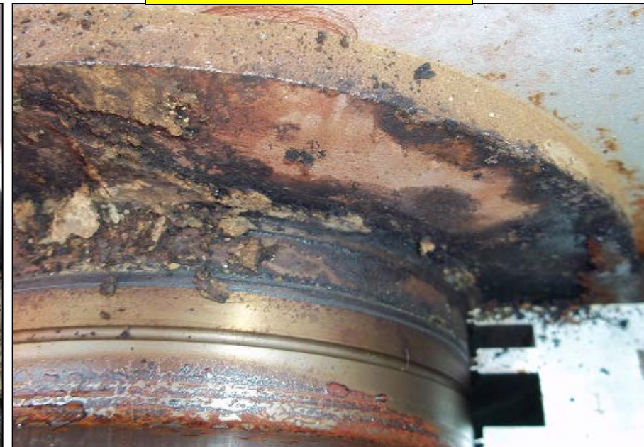
Seal Area of 3 rd Turbine
