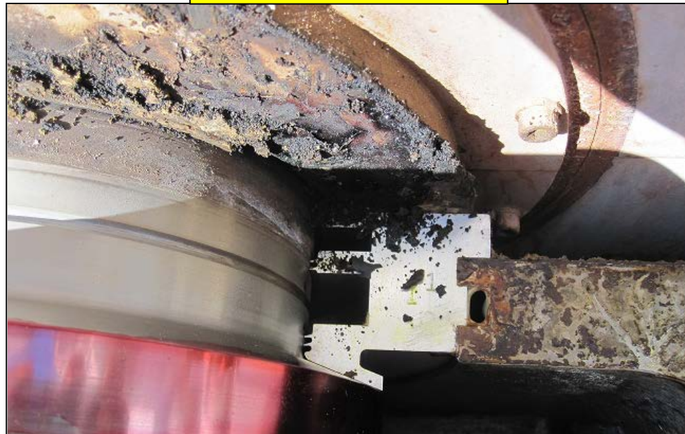
Seal Area of 2 nd Turbine
