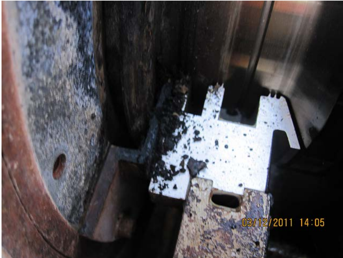
Carbonized deposits at NDE seal area
