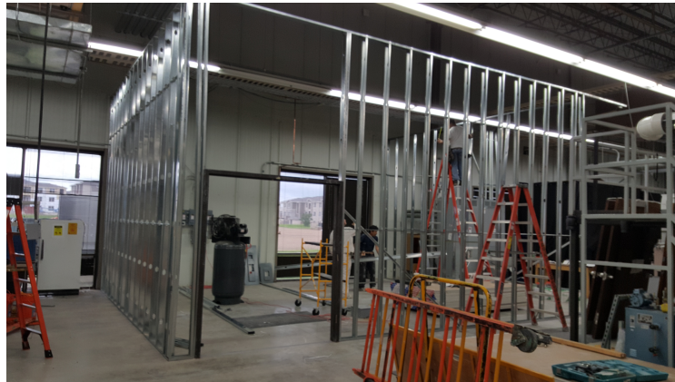
Figure 4.45: Aluminum framing of the facility room
