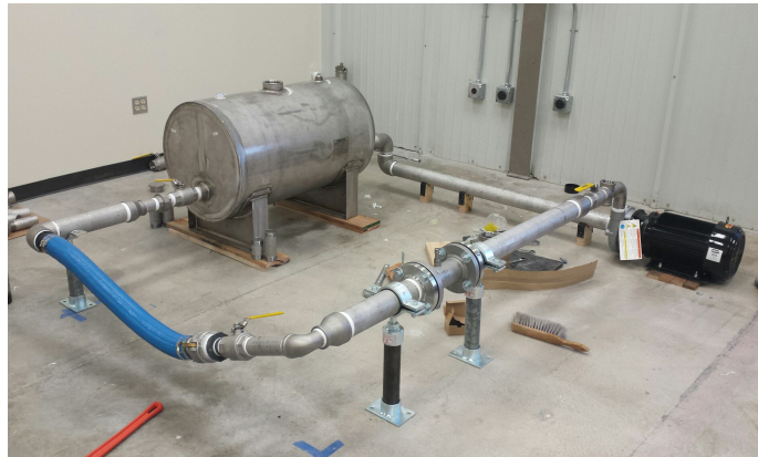
Figure 4.40: Initial leak testing configuration
