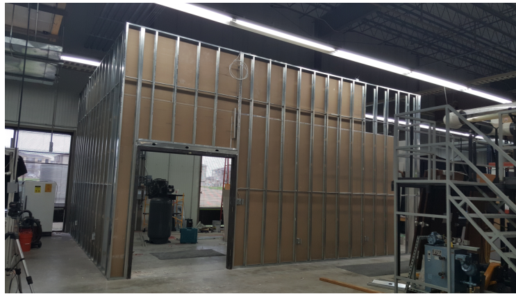
Figure 4.46: Drywall preparation
