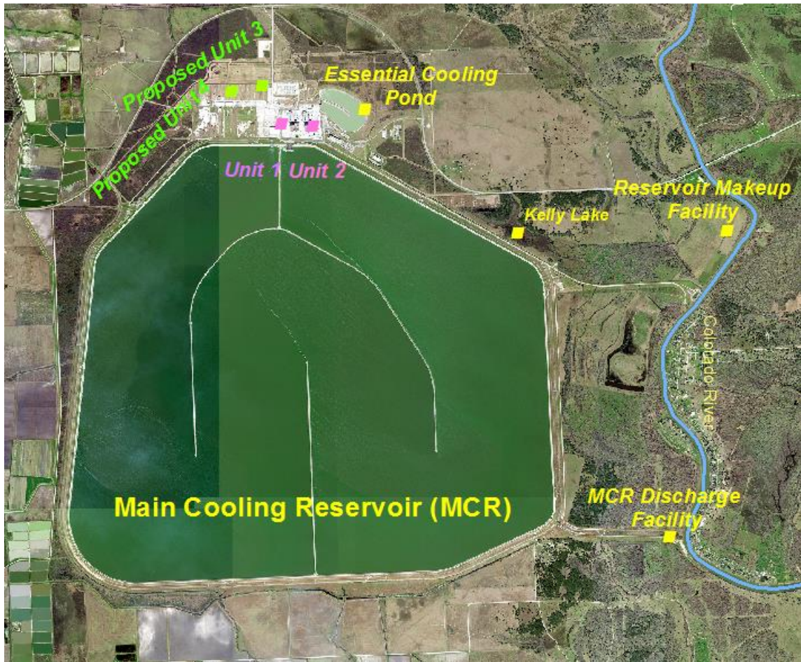
Figure 30. The Sketch of Proposed STP Site (Shapefiles: TNRIS (TNRIS, 2015b), TWDB (TWDB, 2009) )
