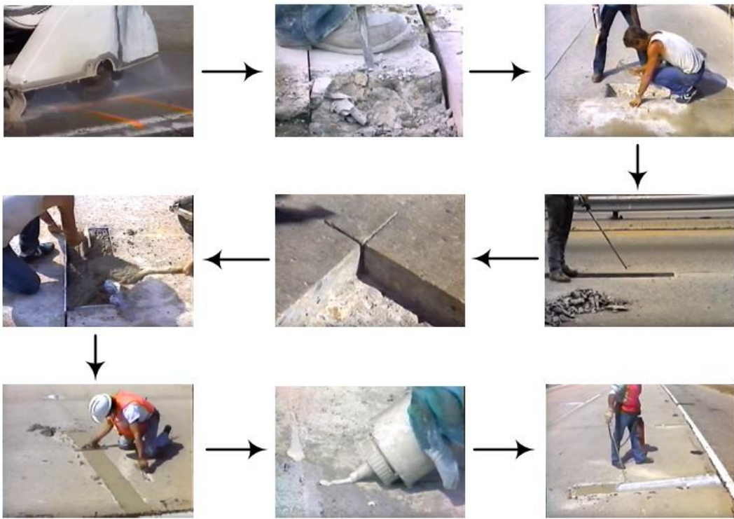
Figure 2 Mill-and-Patch Repair Sequence (FHA 1994)
