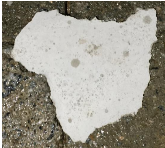
Figure 18 After Gluing the Prefabricated Concrete Segment onto the Spall
