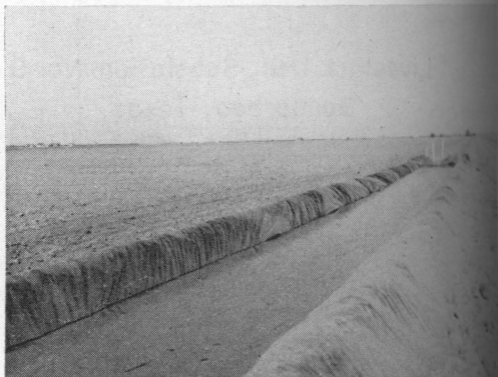
Plastic lining reduces loss of water in irrigation ditches.
