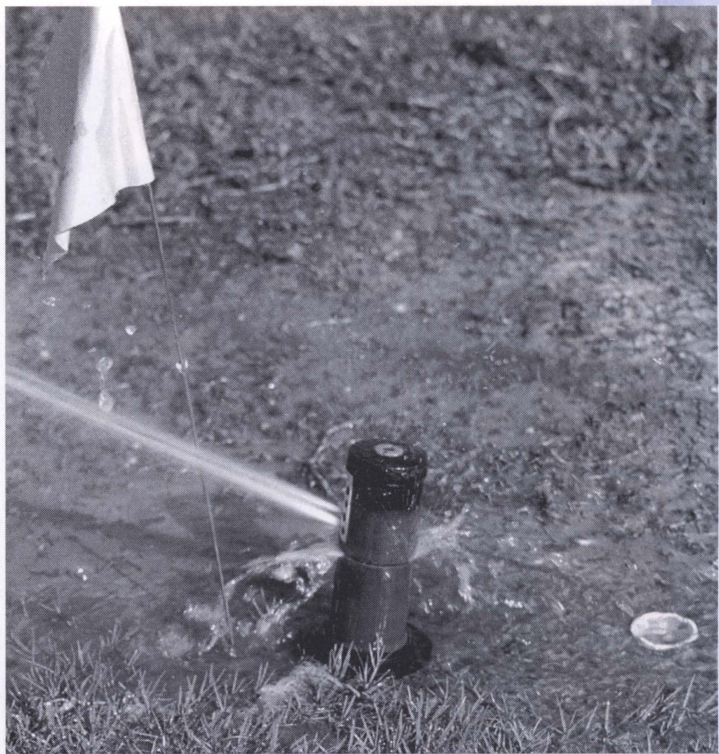
While performing the audit, look for broken or damaged heads.
