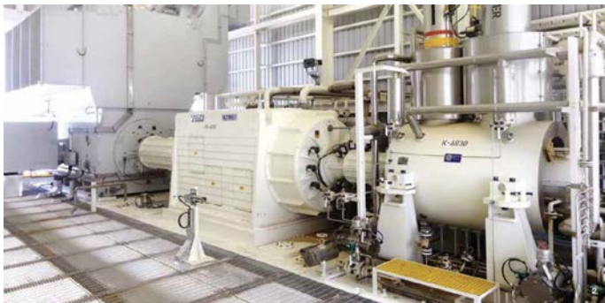
FIGURE 28: ELECTRIC MOTOR DRIVEN CENTRIFUGAL COMPRESSOR WITH INTEGRATED TORQUE CONVERTER AND GEARBOX
