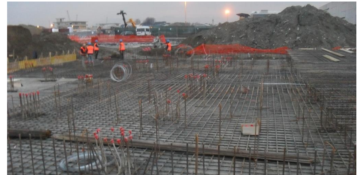
Piles Layout (left) and piled slab under construction (above)
