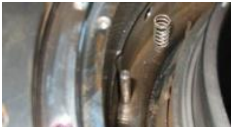
Figure 11: contaminated seal area behind stationary face
