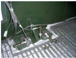
Figure 8: Accelerometers installation on LCC foot
