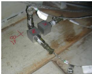
Figure 7: Accelerometers installation on GT supporting girder
