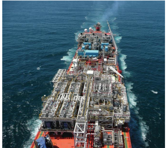
Figure 6. Two 27 MW steam turbine generator sets on board the Knock Allan FPSO for power generation.
