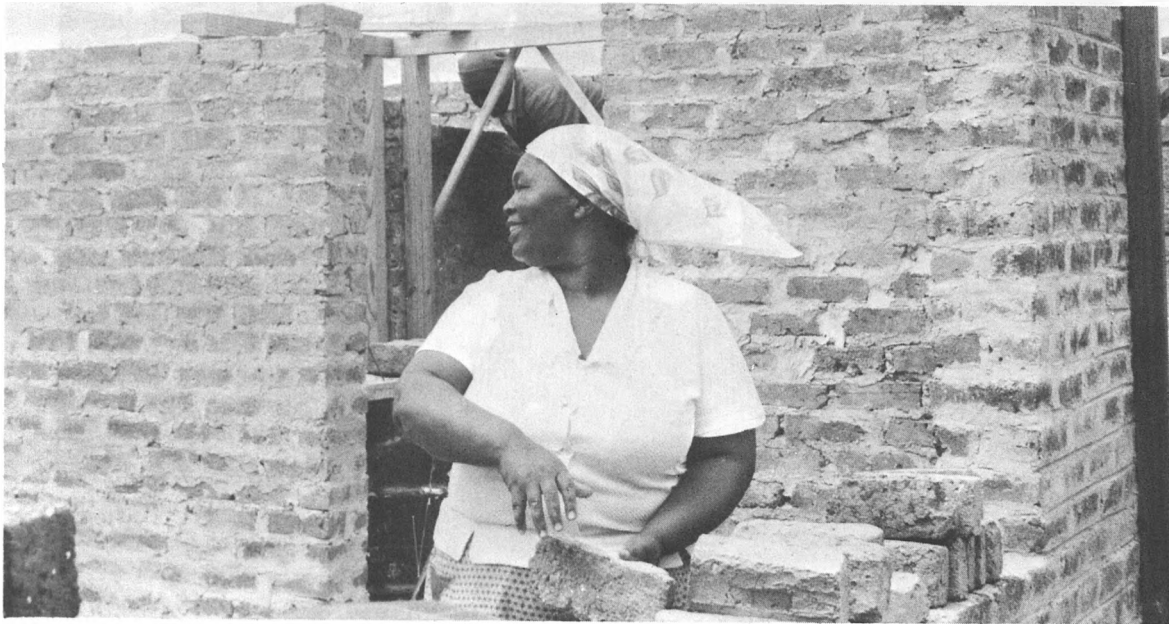
Self help construction
