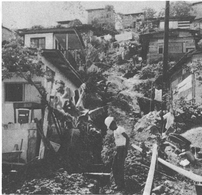
Installation of sewer lines and electric poles in steep hillside
