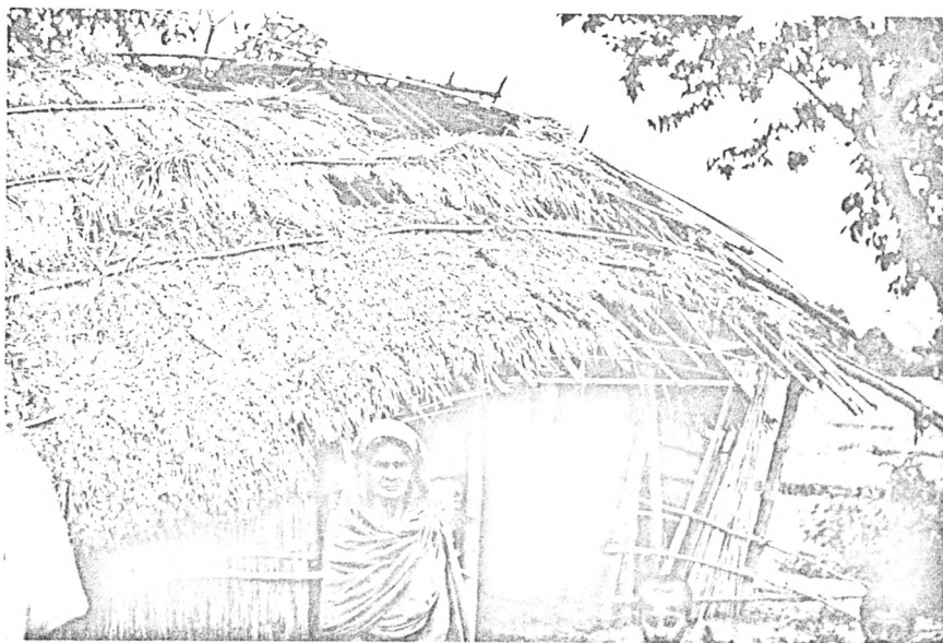
20. Structural as well as roof damage as a result of storm
