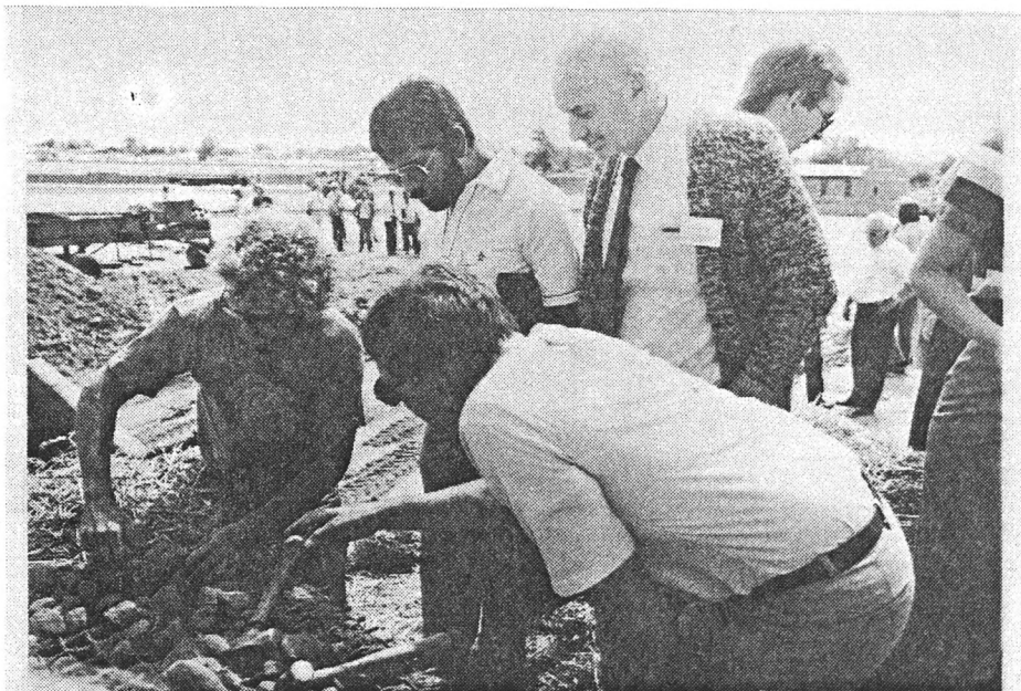
Figure 11. Mixing in the straw at the adobe yard.
