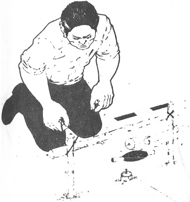
Build a batterboard over each stake.
