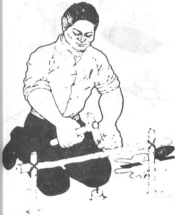
Put a nail in the batterboard at the mark.
