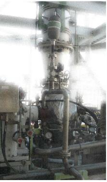
Dampener sized to attenuate pulsations at teeth-frequency (8x running speed; primary excitation measured in field data)
