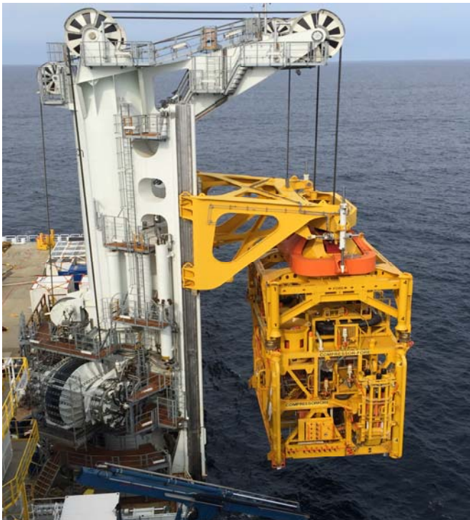
Figure 8: Load-Out of the Subsea Compressor Module into the Norwegian Sea during 2015 (Courtesy of Statoil ASA)
