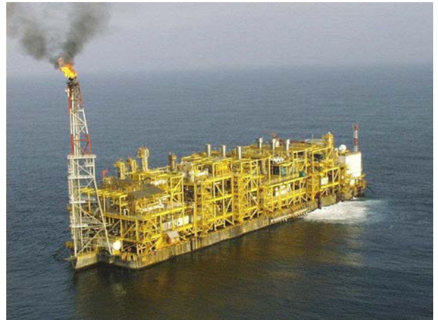
Figure 1: N’Kossa is an oil, gas and condensate field production, located 60 km offshore Pointe-Noire, Congo
