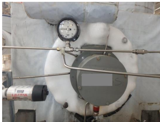
Figure 21: Nitrogen quench – seal area comparatively warmer than the pump
