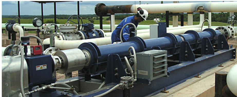
Figure 1.5: ESP in a surface mounted installation. Intermediate supports are used to hold housing in place. [6]
