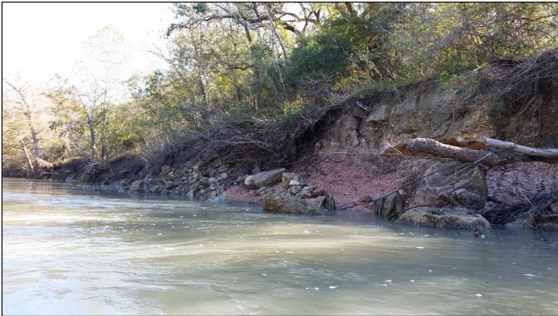
Figure 36. Example of collapsing banks as a result of undercutting. Photo near Cuero, TX. (December 5, 2015).
