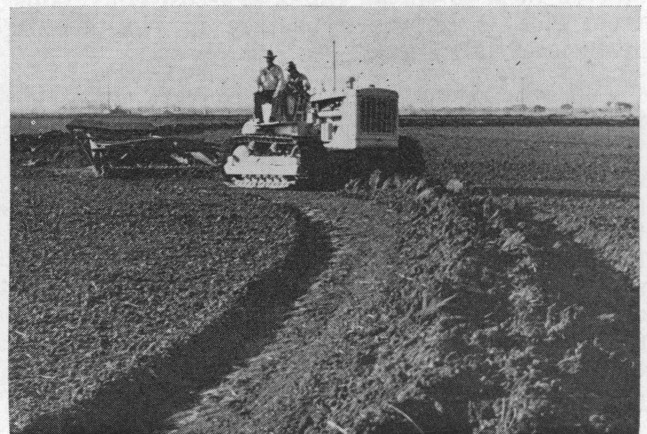
Figure 5. Building levees in a rice field.
